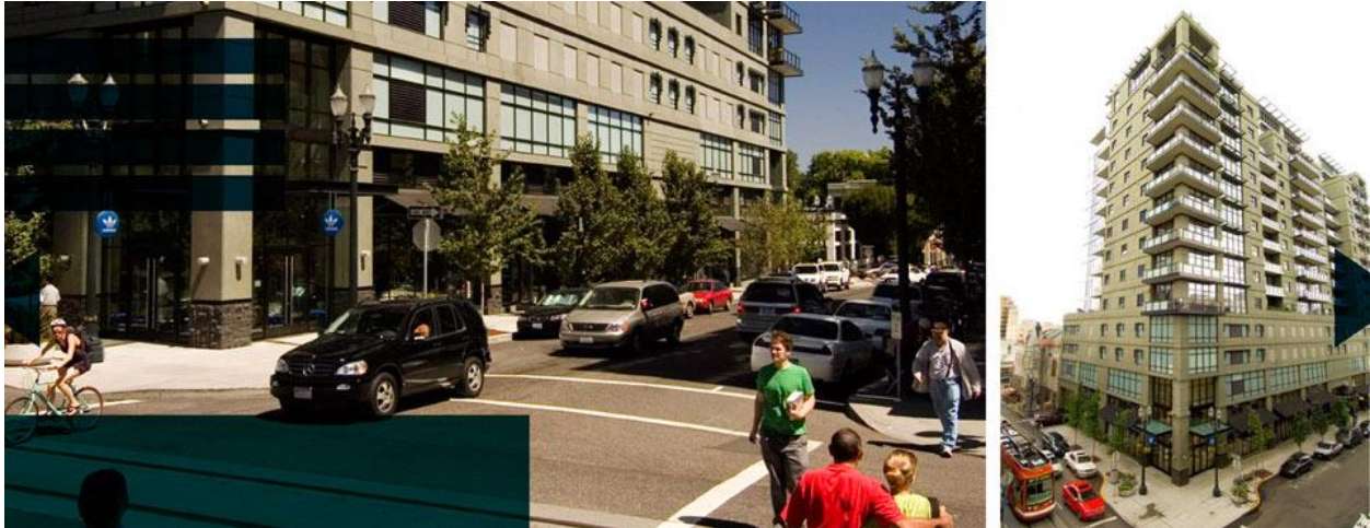
Figure 40: The Henry condominiums in Block 3. 93
