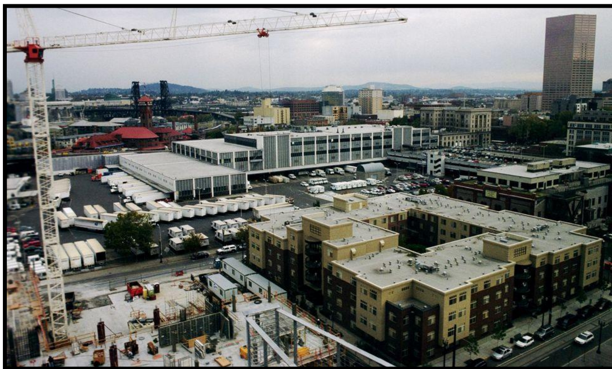
Figure 17: Aerial view of Pearl District Post Office 55
