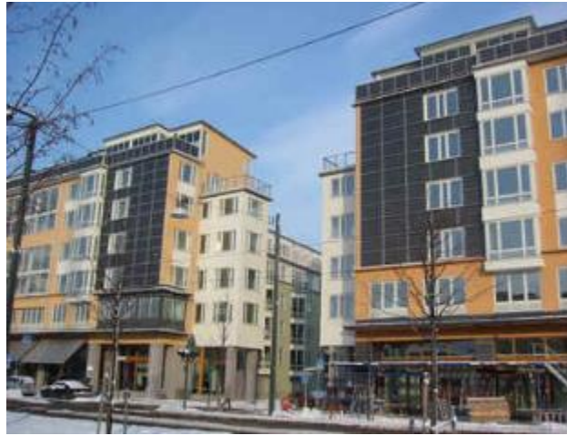
Figure 48. “Holmen” is dominated by the big facades and the long balcony front with solar panels. Source: Solcell.nu
