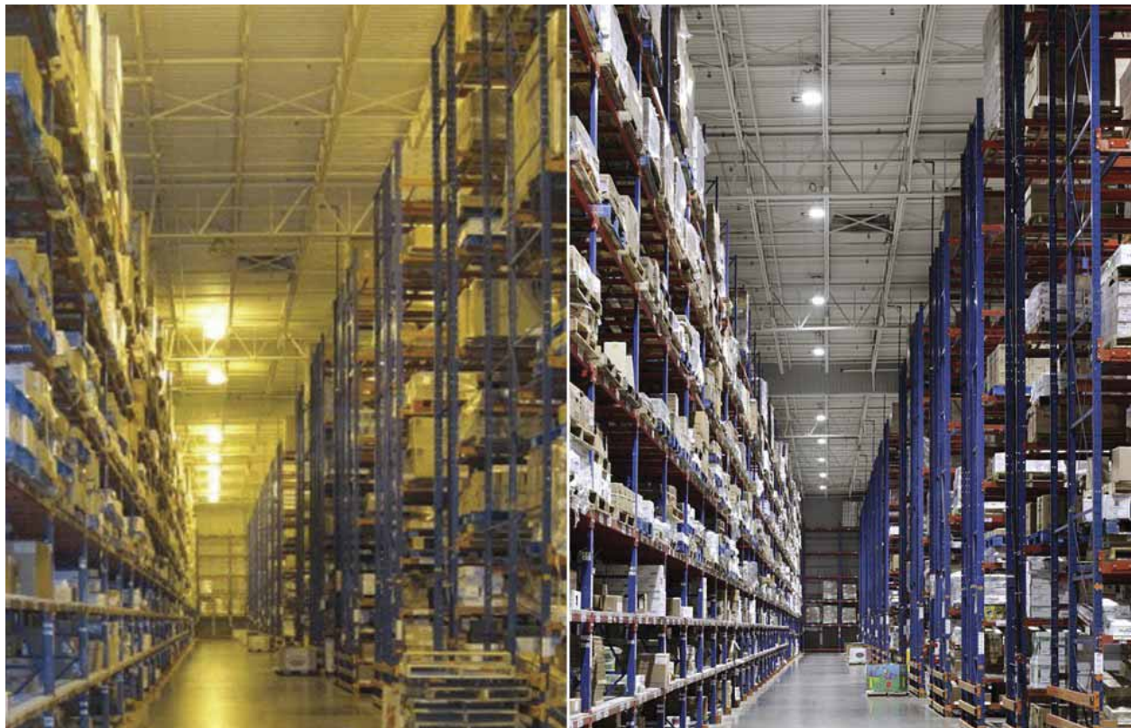
Figure 4-1: Before-and-After Photos of a Digital Lumens Customer Facility
