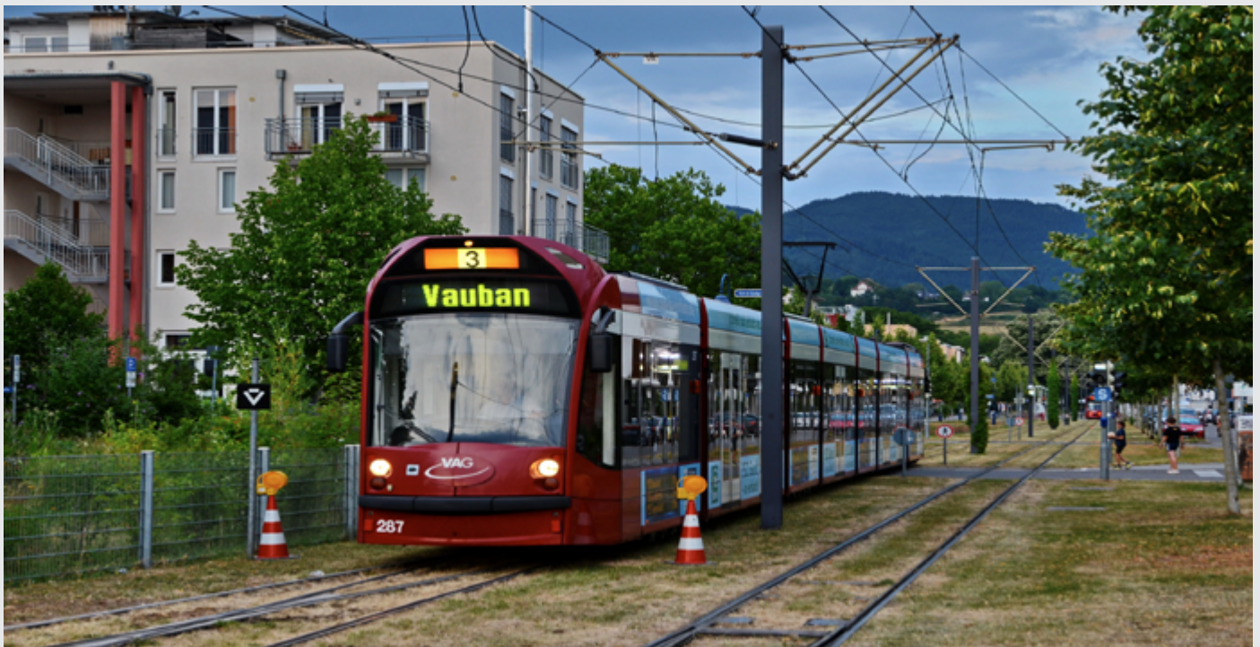
Figure 16. Tram in Vauban with tracks integrated with green space (Source: micagoto / CC BY NC 2.0)
